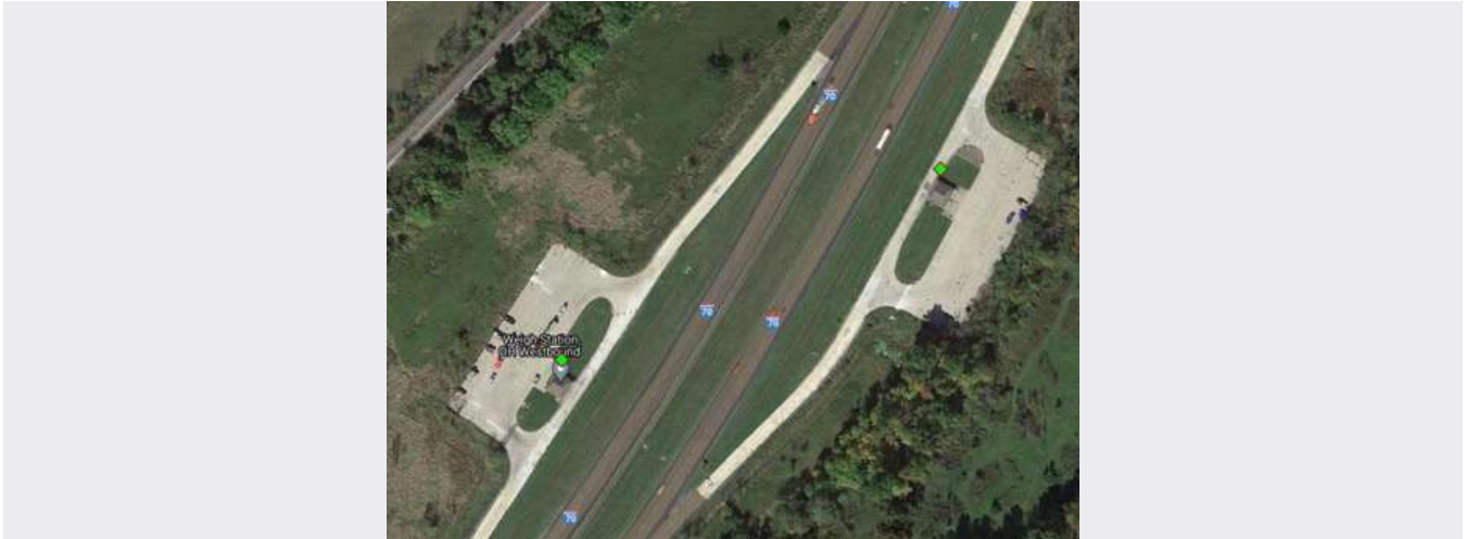
FIGURE 23: OPEN WEIGH STATION ON WB SIDE OF I-70 IN GUERNSEY COUNTY
